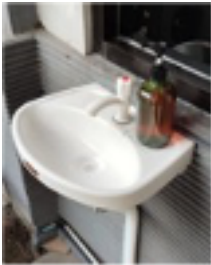
Figure 2. Physical enhancement in the current hand washing facility
